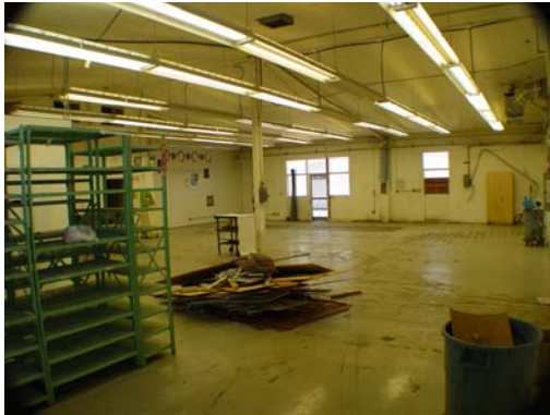
Main Lab Before Renovation
